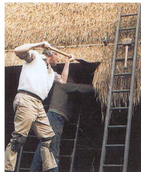
Fig 9 Cutting off a long straw eave
