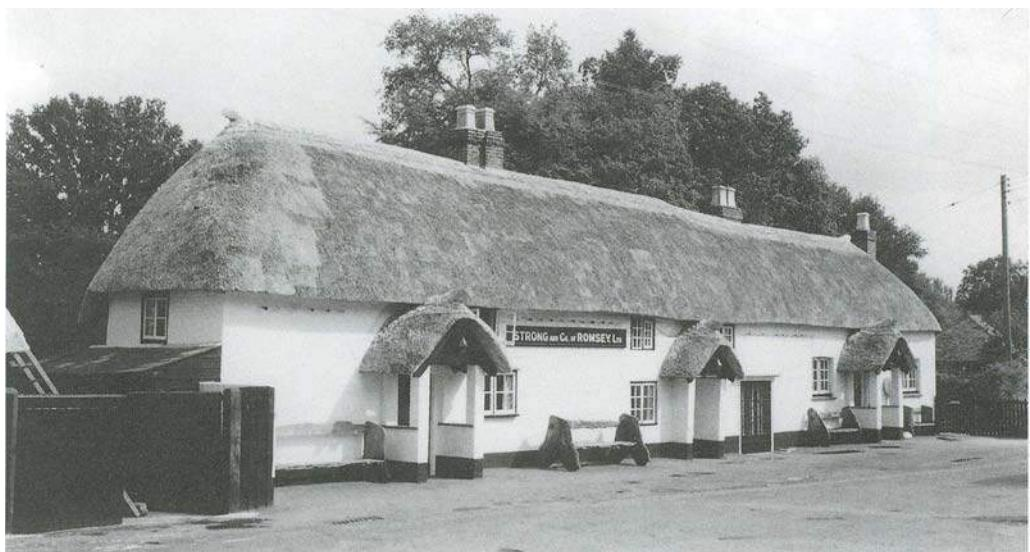
Fig 22 How the character of a building can be affected by re-thatching. The Sir John Barleycorn some years later with a combed wheat reed roof. (Figs 21 and 22 both copyright @ the Rural Development Commission)
