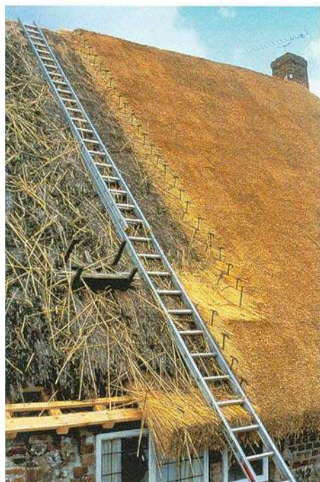
Fig 20 Combed wheat reed being sparrowed onto a pre-existing base of straw. This technique is also used to attach water reed to a straw base. (Photograph copyright © John B Letts)
