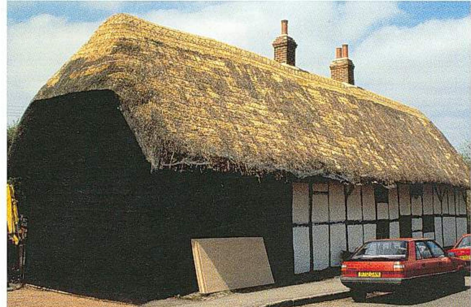
Fig 16 A flush ridge, the treatment which would have been normal in most thatch areas until recently.
